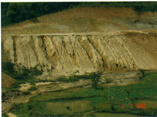
Fig. 1: Erosion on batter during construction in 1988-99. Fig. 2: Vetiver planting in 2000
