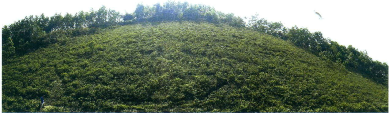
Fig. 4: Panoramic view of the slope full of vetiver Hong Kong Highway Batters and Landslips Kwai Shing Site
