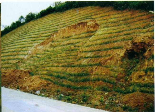
Fig. 1: Erosion on batter during construction in 1988-99. Fig. 2: Vetiver planting in 2000
