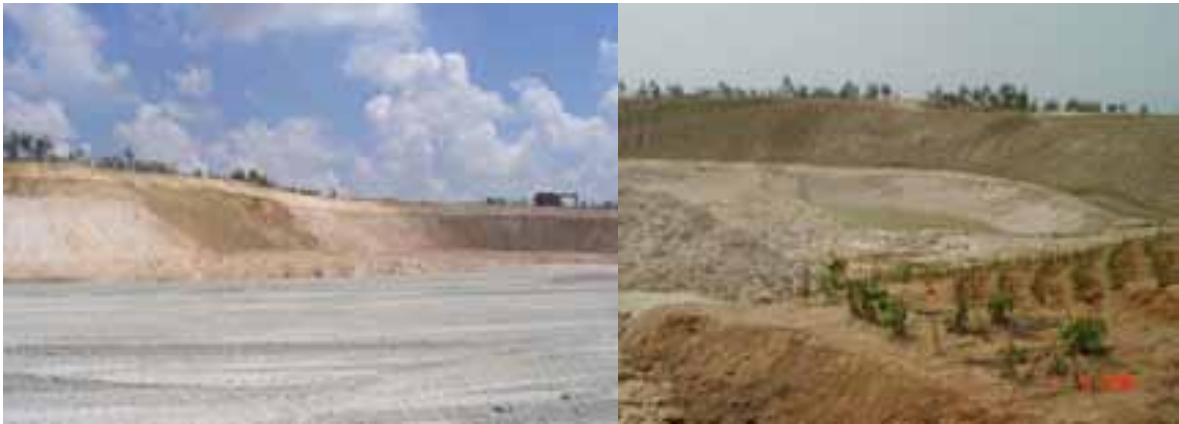
Fig. 11 The largest vetiver project with the area of about 16,000 m 2 Left: parts of the panorama prior to planting vetiver. The white parts are all kaolin Right: the landscape that vetiver was just planted on the slope
