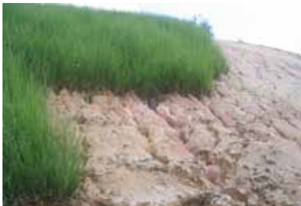
Fig.13 A contrast for erosion control and slope stabilization with or without Karnataka vetiver
