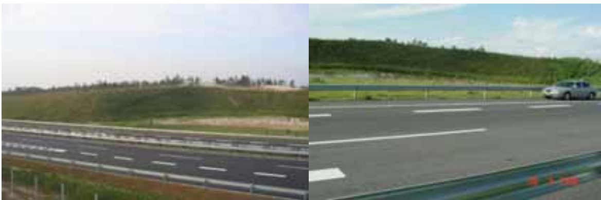
Fig.12 The landscape of the largest cut after Karnataka vetiver was planted for two months (left) and for eight months (right)
