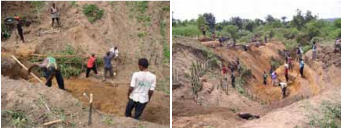
Photo 4: Retaining barriers built with tree branches
