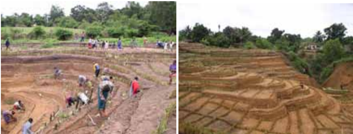
Photo 5: Planting vetiver hedges on contour lines on the terraces
