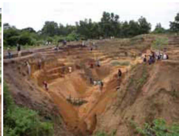
Re-profiling the slopes of ravine ITPKA
