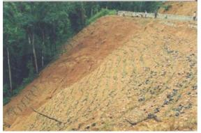
Fig.16 Shallow seated failure of embankment Fig.17 Repair of the collapse embankment slope at STA.15+325-STA.15+510L before stabilized by vetiver.
