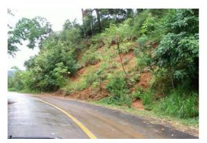
Fig.4 Erosion and shallow seated failure on highway cut slope
