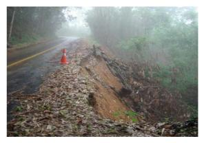
Fig.5 Shallow seated failure on highway embankment slope
