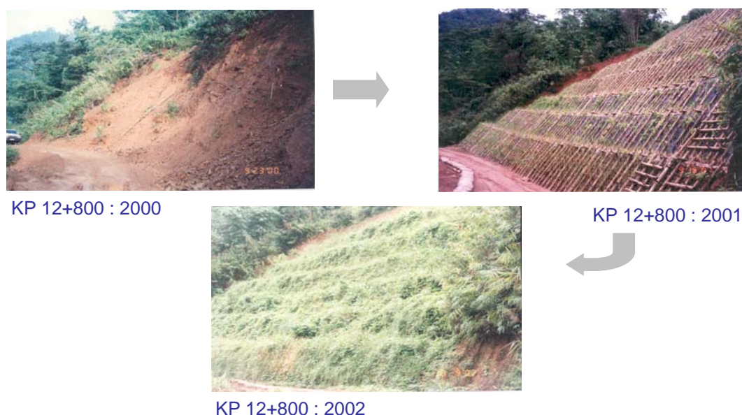
Figure 10 : KP 12+800, The application of jute sacks and vetiver grass were used for stabilize steep shoulder slope.
