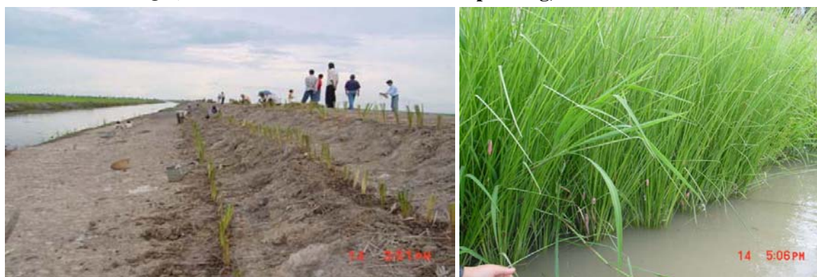
Photo 4: Left, Vetiver grass planted on a dyke at the experimental site in Tri Ton Right, well established after the second planting, six months later
