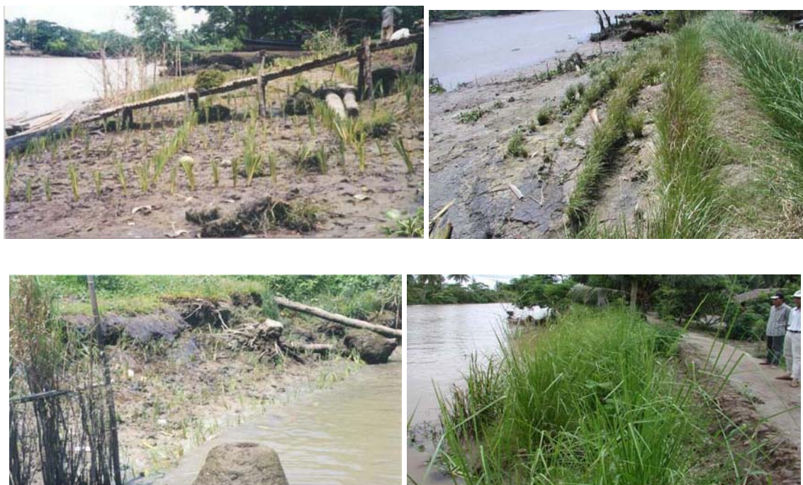
Photo 5. Left, Newly planted on an eroded site and Right, 8 months later
