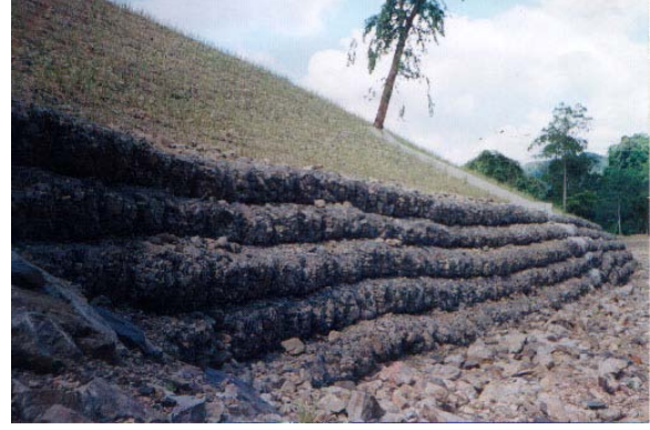
Fig.19 VS is associate with gabion wall in the rehabilitation work on Highway Route No 1451: Sec. Adj. to Phattalung Highway District's Area – JRT.Highway No. 403.
