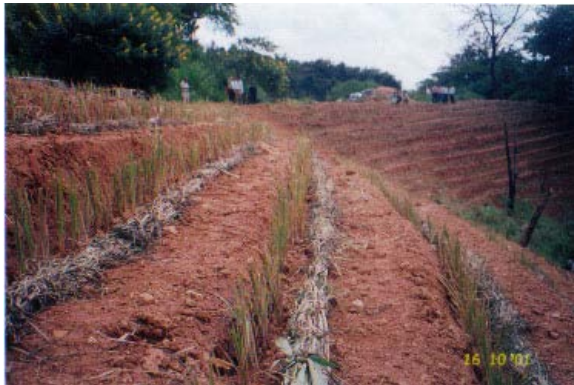
Fig. 13.1 Repair of the collapsed embankment slope in Fig.4 and stabilized with vetiver.
