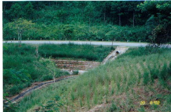
Fig. 13.2 Embankment slope was stabilized with vetiver for 1 year.
