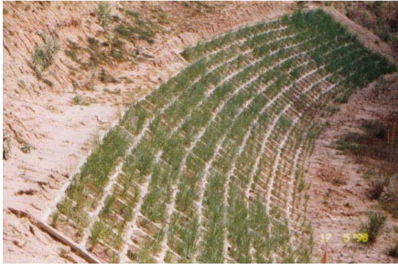
Fig.18 VS is applied with concrete square grid slope protection in the rehabilitation work on Route No.108: Hot – Mae Saring.
