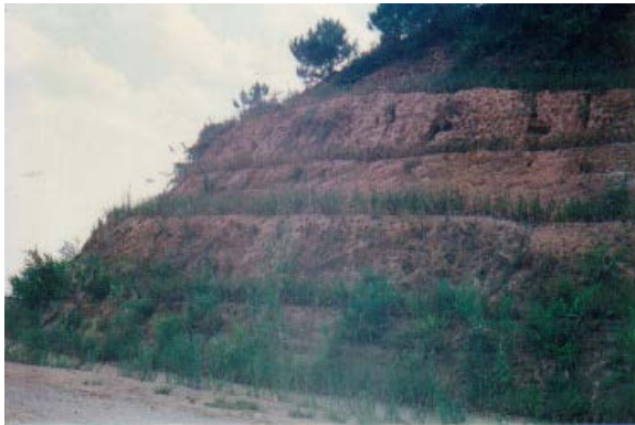
Fig.11 Highway cut slope was stabilized with vetiver on Highway.
