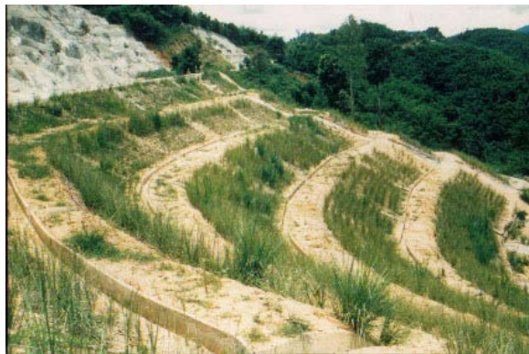
Fig. 14 High embankment was stabilized with vetiver coupled with surface drainage systems in the rehabilitation on Highway Route No.109: Fang – Tha Thon
