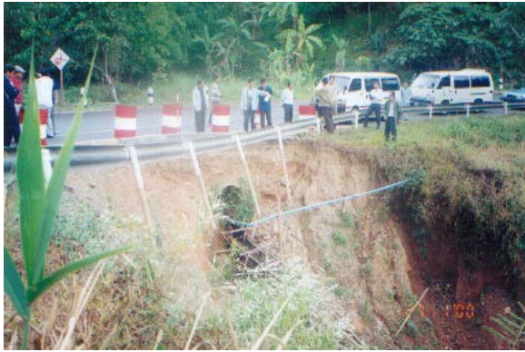
Fig. 4 Erosion at the end of pipe culvert and drain chute.
