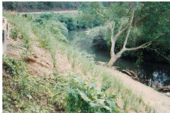
Fig.15 Stabilization with vetiver along the stream bank on Highway Route No.107: Ban Pingkoke – Saphan Huai Tai.
