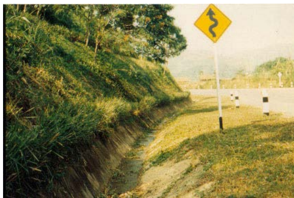
Fig. 16 Vetiver planting at the side ditch lining.
