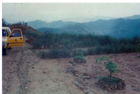
Fig. 17 Vetiver planting on highway shoulder to slow down runoff longitudinal.
