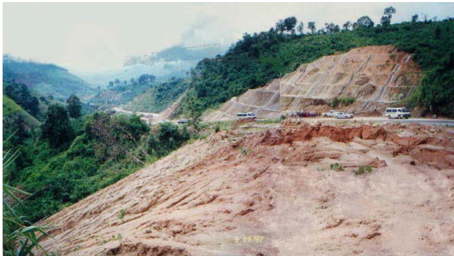
Fig.6 Highly erosion of uncompacted sandy soils on surface of embankment slope.
