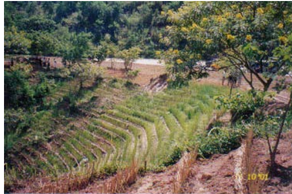
Fig.12 Highway embankment was stabilized with vetiver on Highway Route No.1149:
