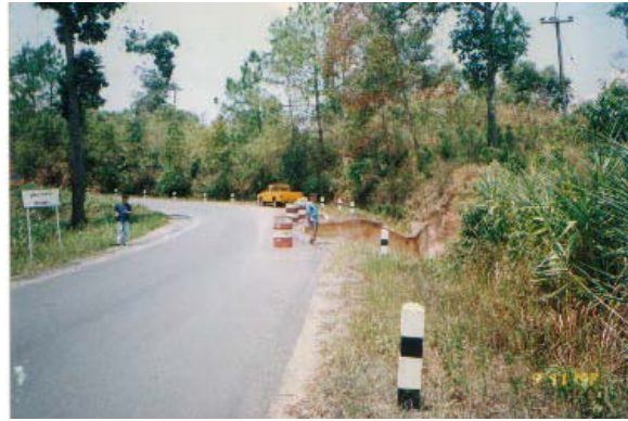
Fig.5 Large gully erosion caused by the erosion at the end of side ditch.
