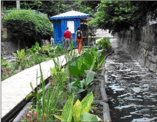
Photo 1. Hydroponic treatment of sewage with other plants
